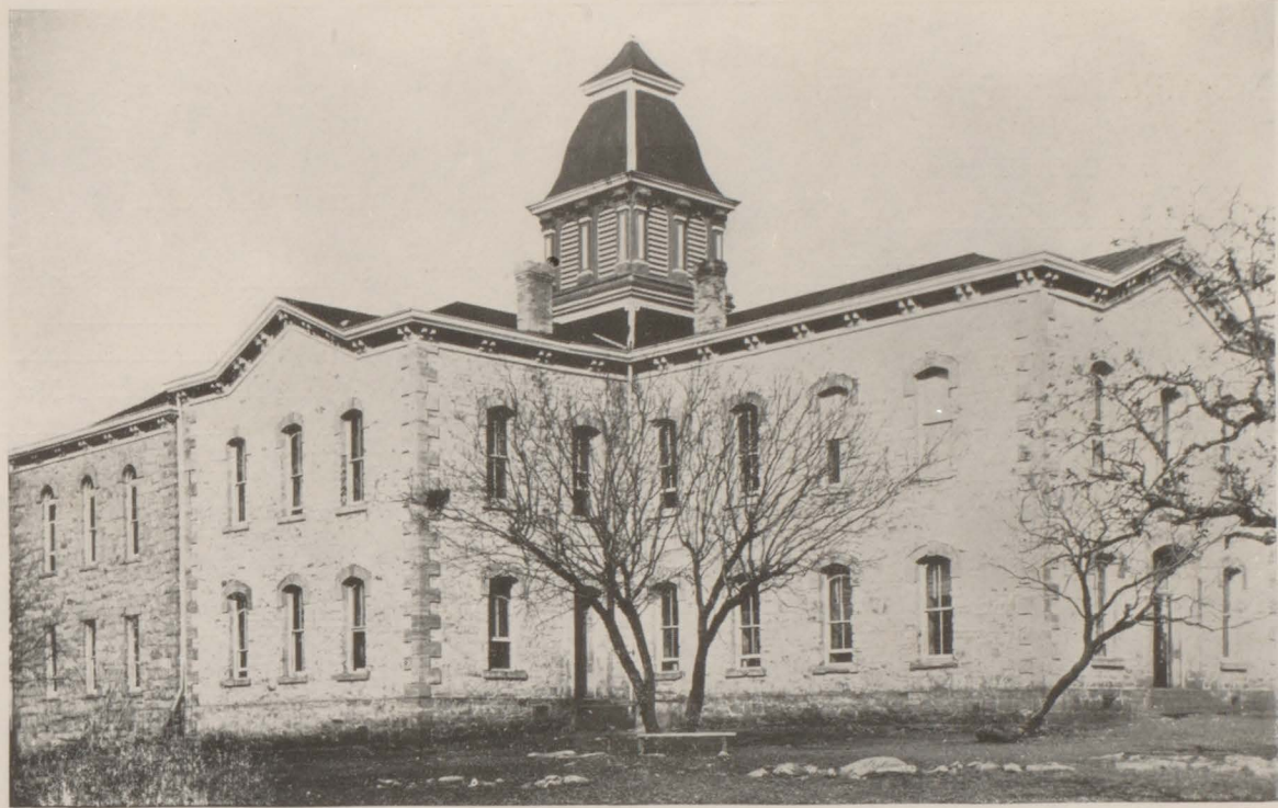
Llano High School Building
