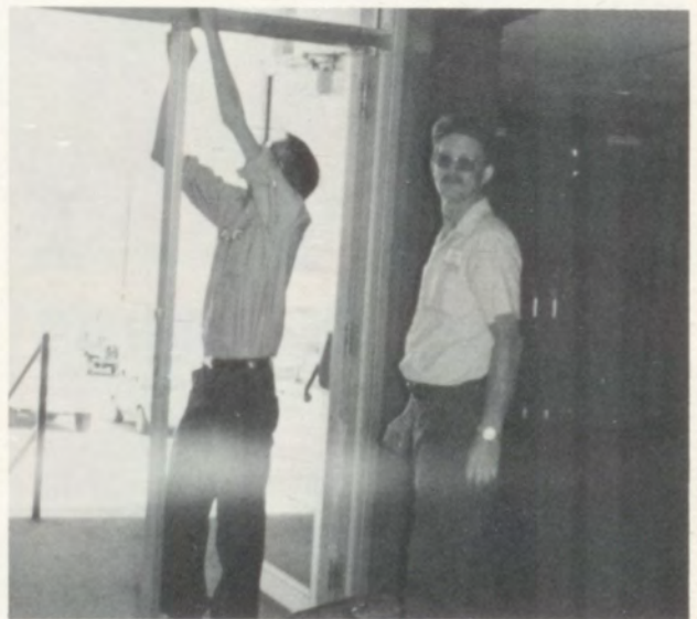
MR. WADE and MR. HENSLEY repair a broken door.
