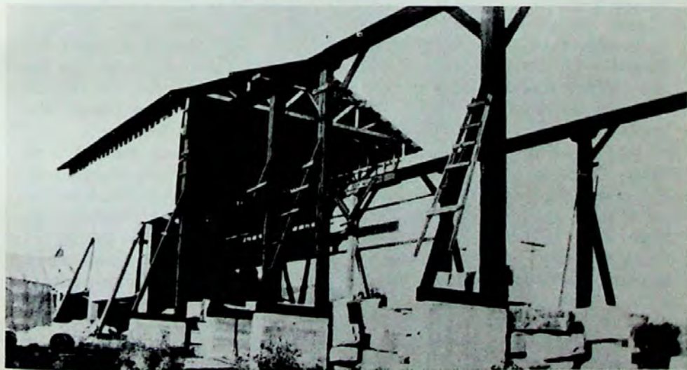
One of the derricks that were used to load and unload granite.
